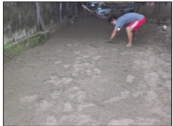
Leveling the sand and gravel
