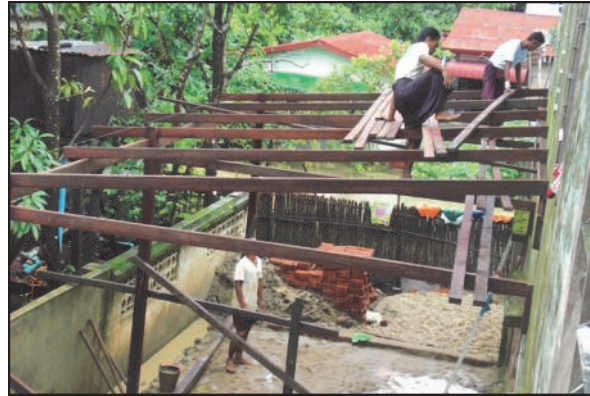
Building the side addition for HBS
