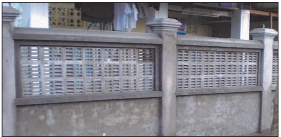
The front fence under construction
