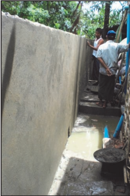
Building the back fence for HBS
