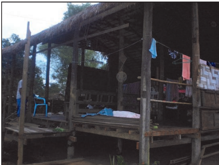
Pastor Lun Kho Thang's current house. Note the lack of walls on three sides.
