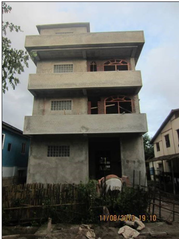
The completed shell of the new building
