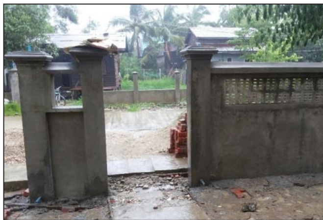
A portion of the new front security fence under construction
