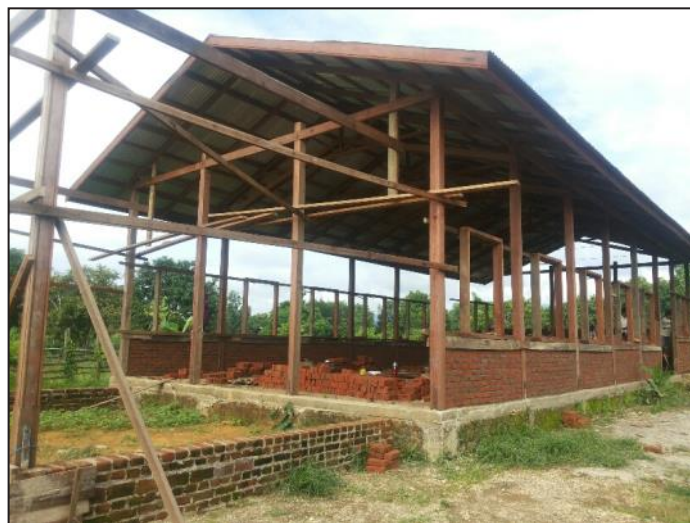
Namihan Christian Church under construction
