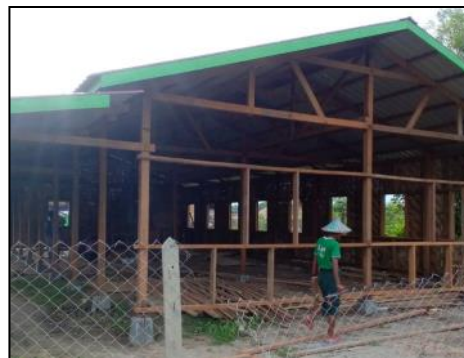
School building under construction
