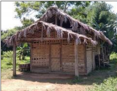
Shwepyita Christian Church—Old Building
