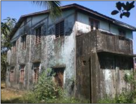
The original HBS building in 2010
