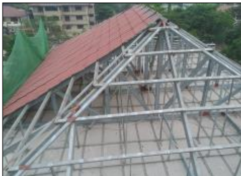
Replacing the roof on the Girls' Dorm
